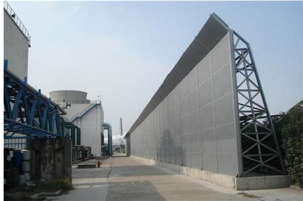
Cooling tower with sound insulation
