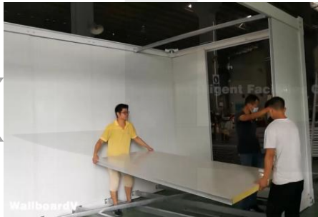
7. Install wall panels
