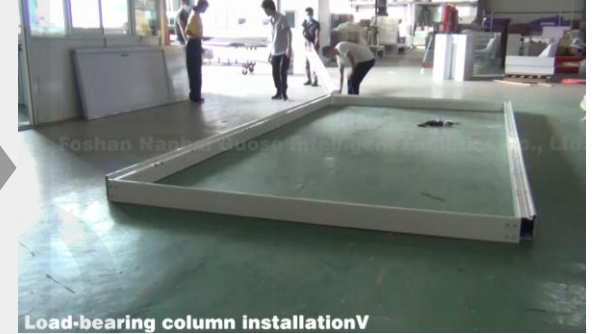
4. On-site assembly, placing the bottom steel beam
