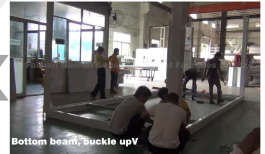
5. Install the column and the bottom tube
