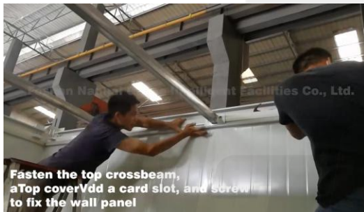
9. Install the top square pass
