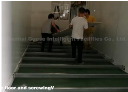
8. Install the floor
