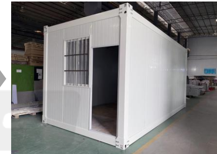
11. Installation is complete
